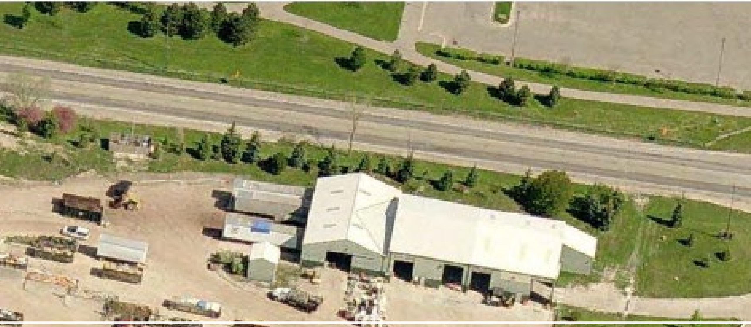
Existing Facility: Ann Arbor Drop-off Station
